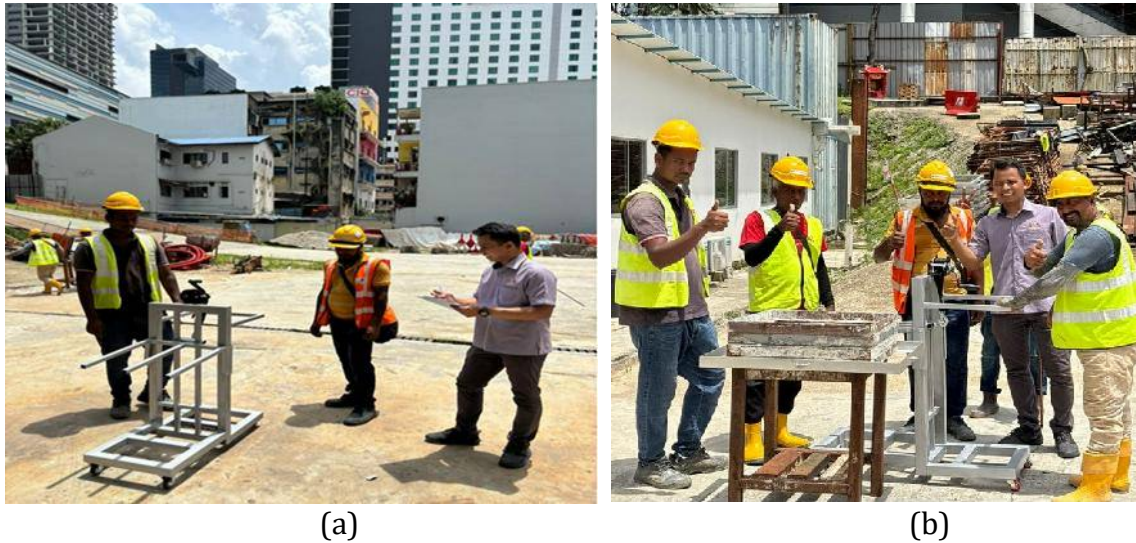
Figure 3: Testing the Smart Mini Portable Lifter at construction site
